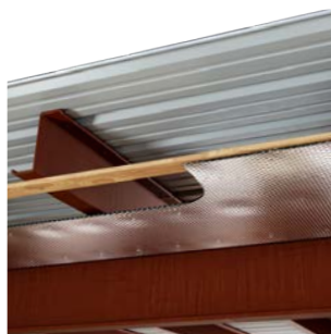
Roof / Retro* R-11 Heat Flow Down R-4.4 Heat Flow Up
