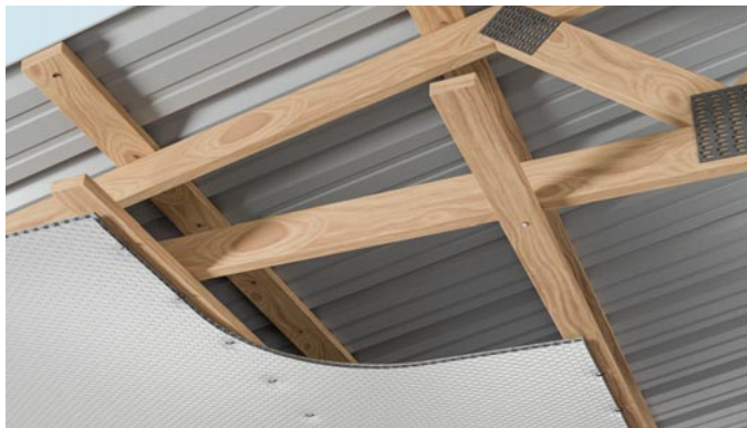
Roof / Retro* R-6.6 Heat Flow Down · R-3.0 Heat Flow Up
